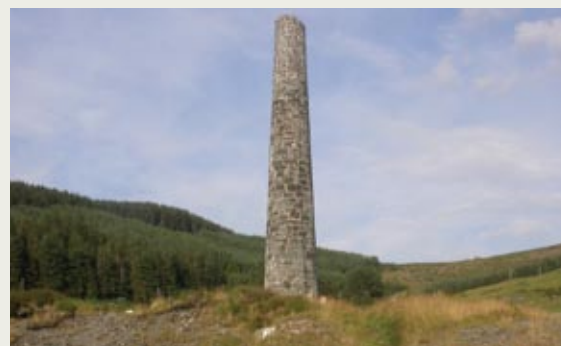
Close cooperation between builders and lichenologists has led to the sensitive restoration of this chimney at Cwmsymlog Mine, Ceredigion
